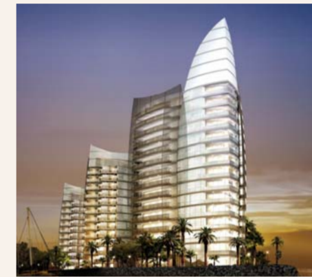
The Oceanfront @ Sentosa Cove Jointly developed by: TID Pte Ltd & City Developments Limited
